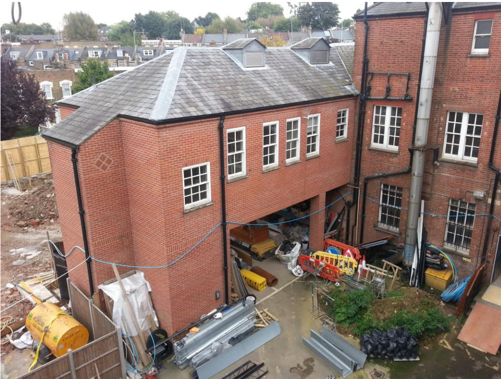
Image 3. View of rear projection from main building
