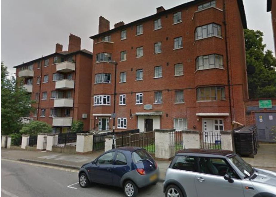
Image 2: View of Kingsley House and Phillips House along Anson Road
